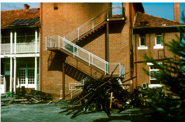
Charred remains shown from the back of the school.
